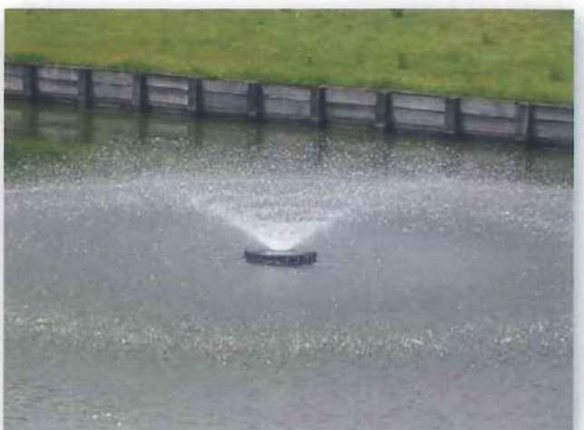
Works.06 | 噴水工事
